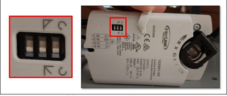
**Modulating Actuator DIP Switches with Correct Settings**
